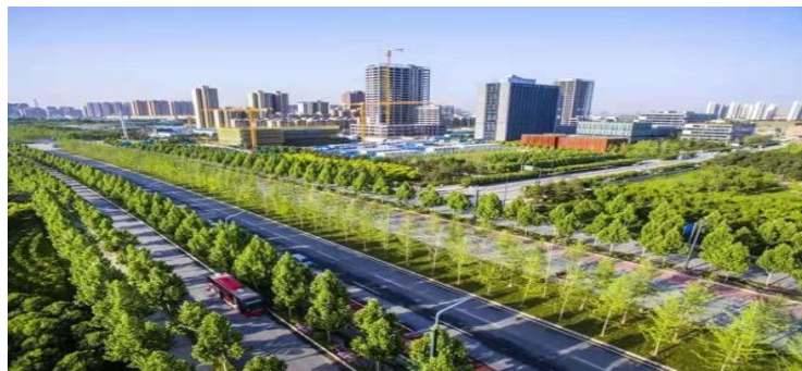
Figure 30. Fengxi New City Case Study. View.
